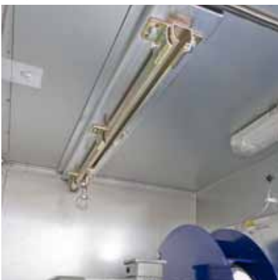
exit rail for replacing the fans
