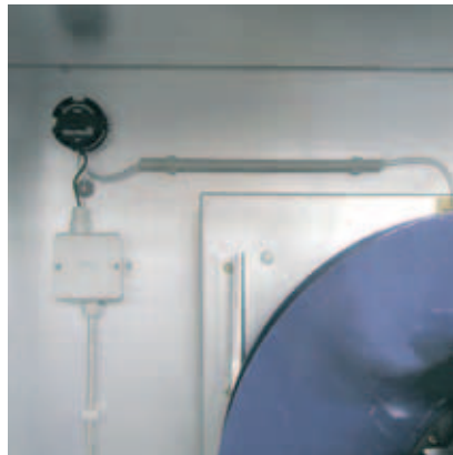
volume flow measuring at the fan
