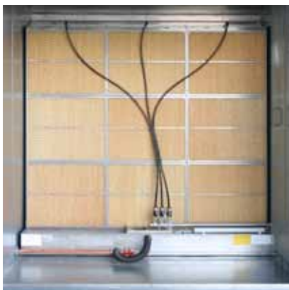
Contact humidifier with three cascades
