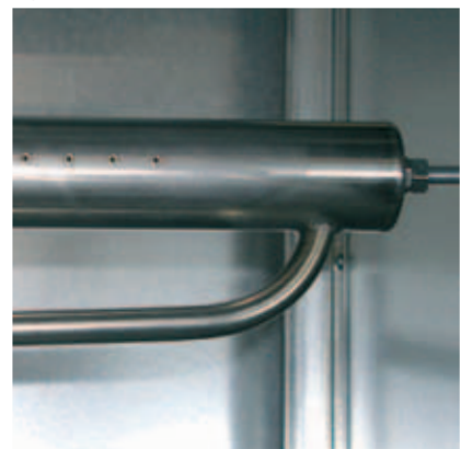
vapour humidifier lance with condensate pipe
