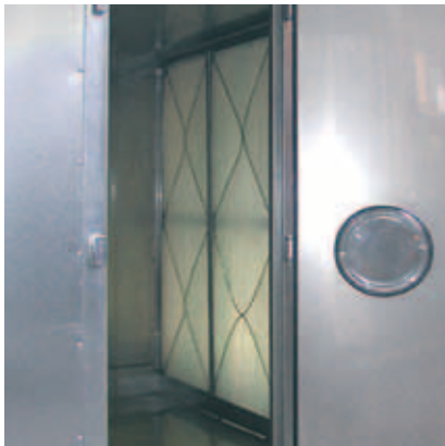
drop separator for high-pressure humidifier
