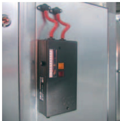
differential pressure manometer (filter supervision)
